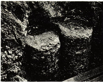
Fig. 16. Lime columns with a diameter of 0.5m
