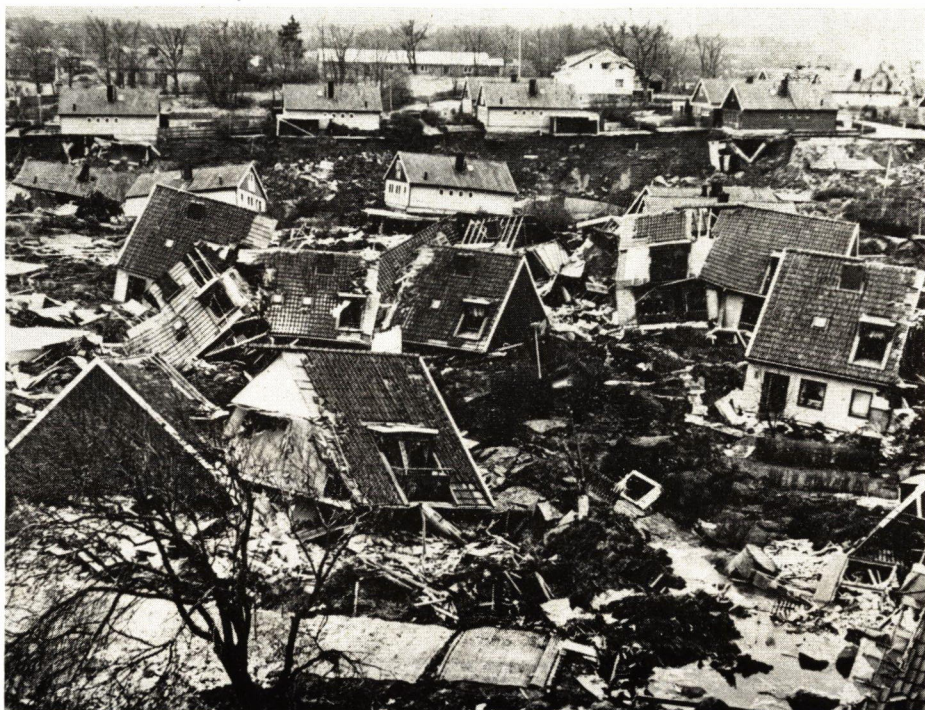
Fig. 4. The total damage costs for the landslide are estimated to be about 140 million Swedish crowns
