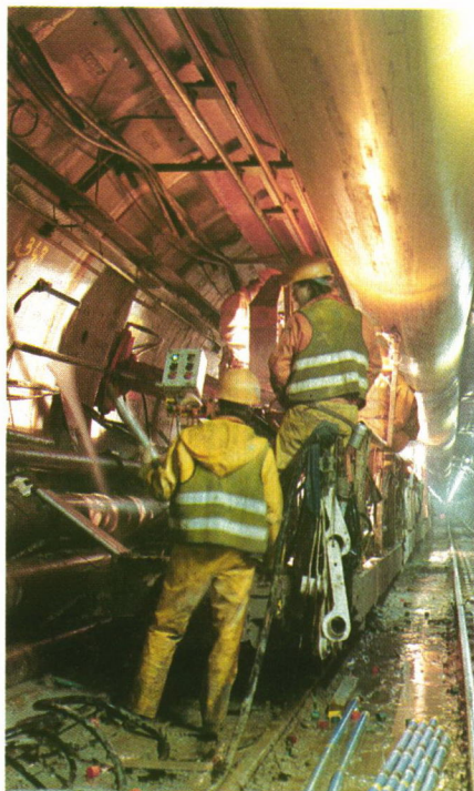
Picture 1: Drilling train in the service tunnel.
