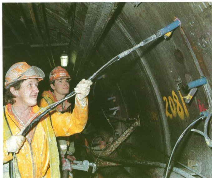
34 Picture 2: Inserting a tube à manchette PCC lined section.
