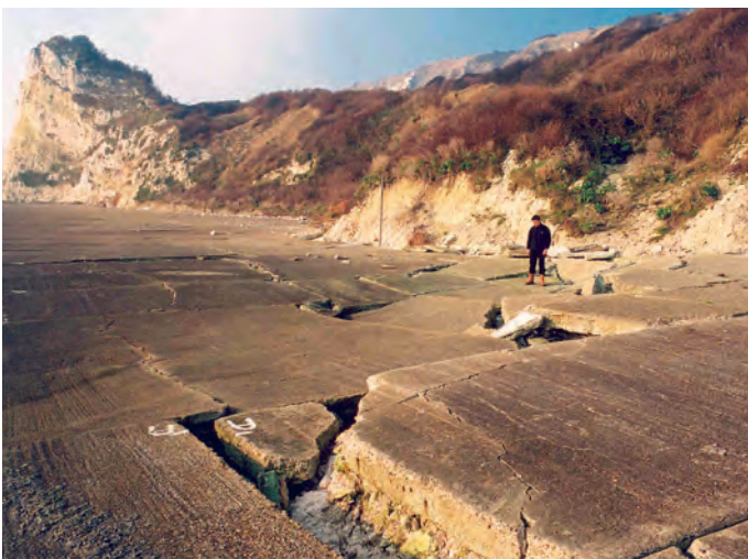
Figure 3: Severed concrete apron at Horsehead Point in 2001
