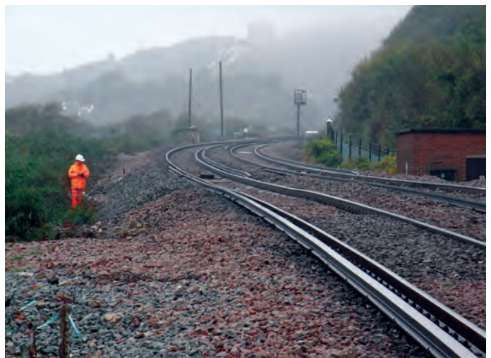
Figure 4: Track distortion at Warren Halt in 2010
