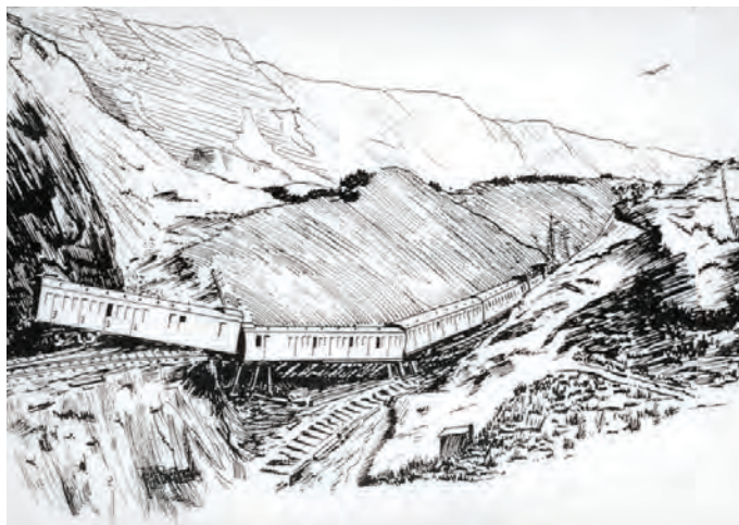
Figure 1: View east of the major slip in 1915
