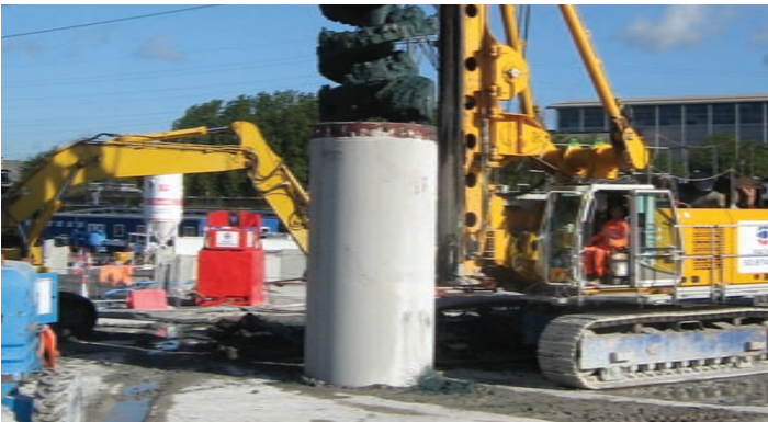
Testing: 80 cores were taken to prepare for construction of the drive shaft
