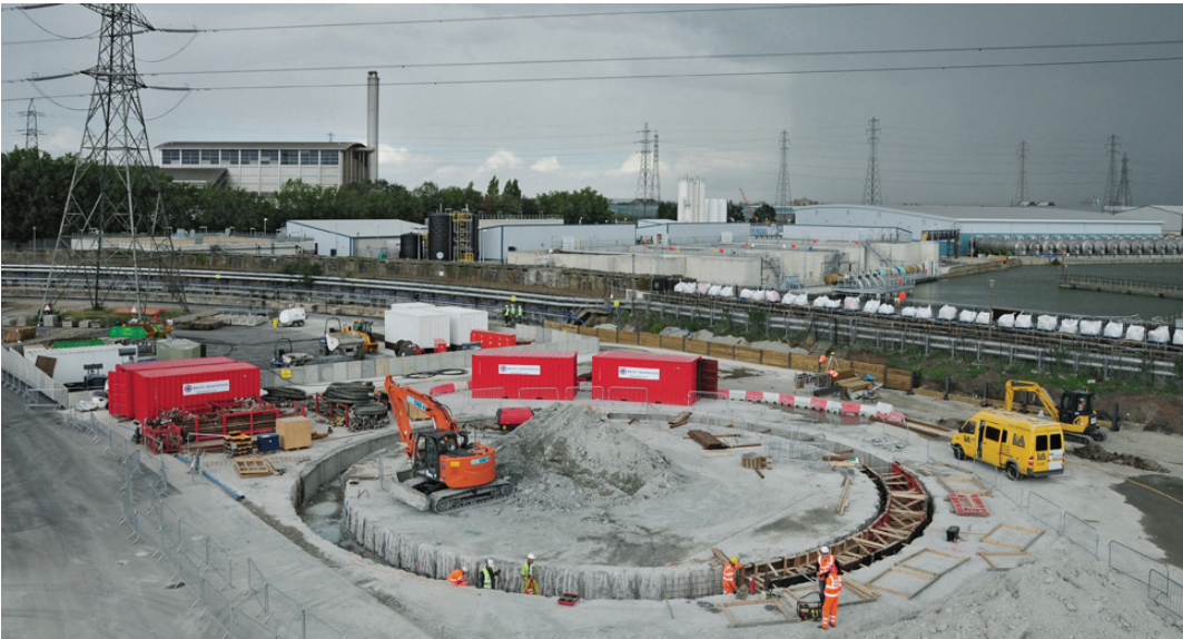
Getting going: MVB will start work on three of the four deep shafts that will be built for the project in 2010
