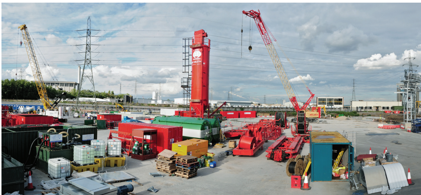
Big spend: Construction is already underway on the Lee Tunnel Project
